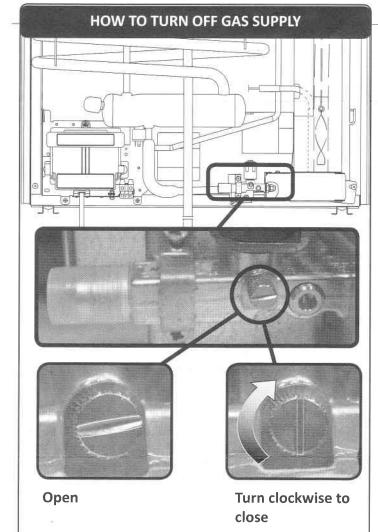
The manual gas valve is located at the back of your refrigerator near the floor as seen in the diagram above. Access the back of your refrigerator by removing the vent on the side of your coach.
